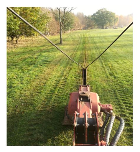
Once the new position of the Irrigation head has been approved by the Irrigation designer we "Hope" that we can "mole plough" the pipe and cable into the ground from the mainline to the sprinkler location.
